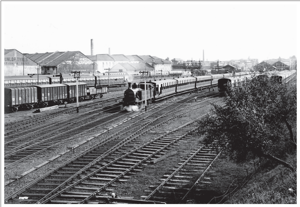
Colaba Station Yard
