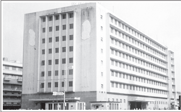
New Churchgate Station
