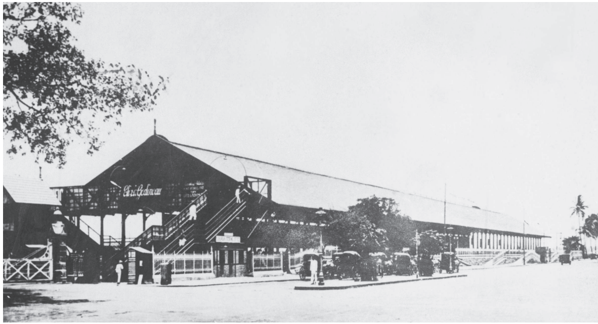
Churchgate Station after Electrification
