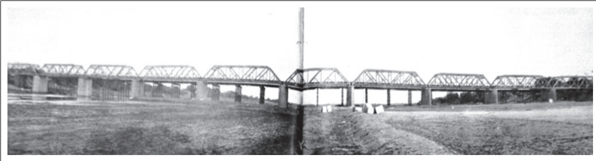
Tapti Bridge consisting of ten 187'-6" Spans
