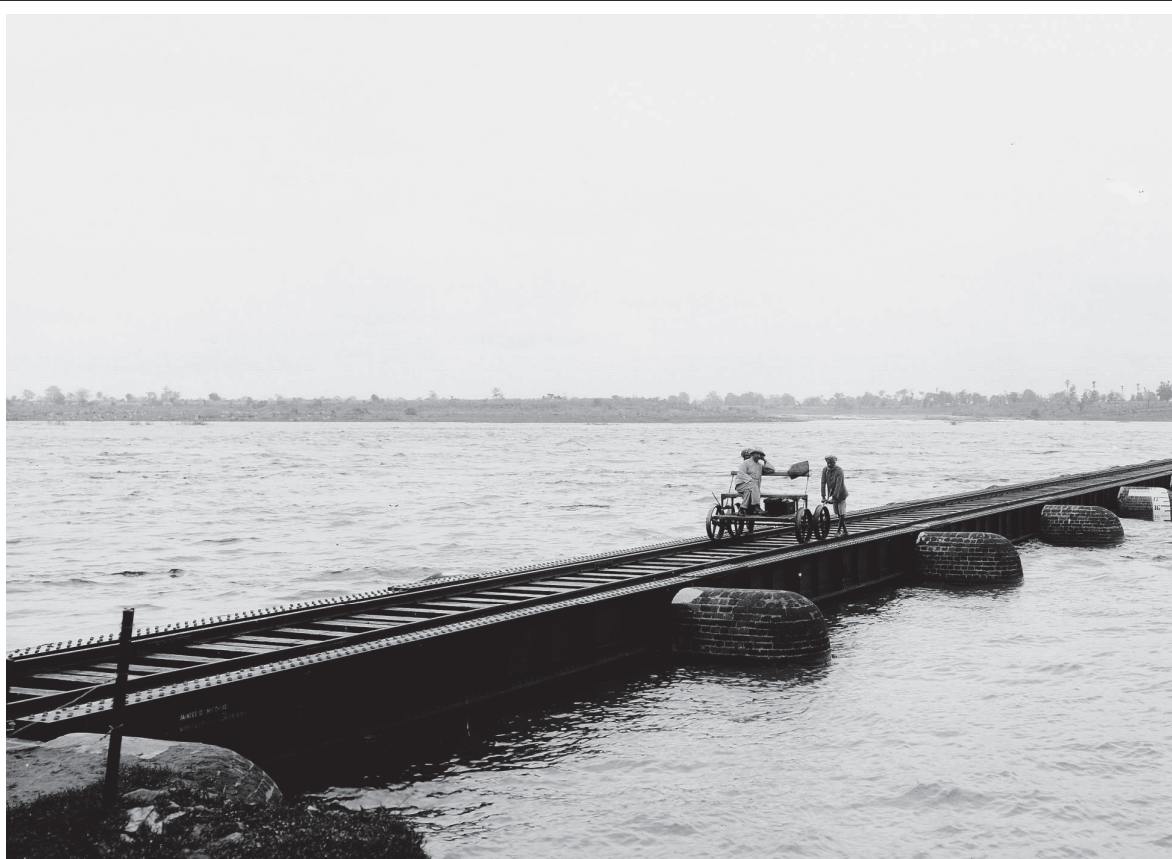
Mahi Bridge at Sevalia
