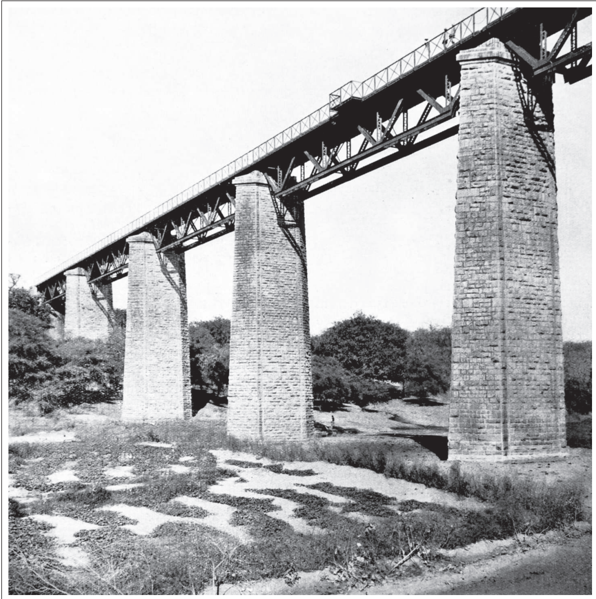
Balaram Bridge MG
