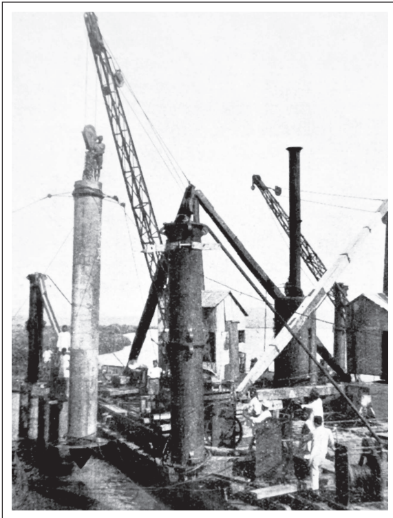
Rebuilding Bassein Bridge: The Pile Screw Capstan at work
