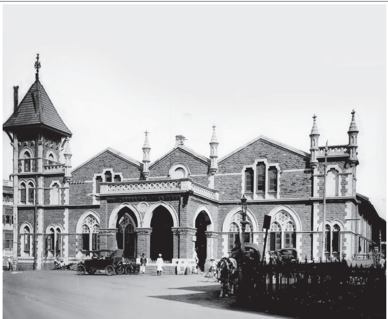
Old Colaba Station, 1896 - 1930.
