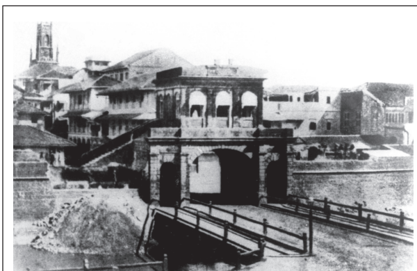
The inner Church Gate Photograph taken when the demolition of the Fort walls had just begun.
